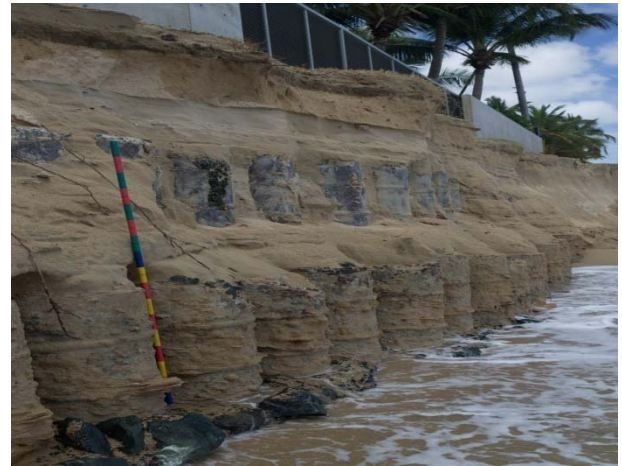
Figure 6. Exposure of informal coastal mitigation structures (Jacob's staff with 10-cm intervals). These containers were used to fill in from 1930 to 1940. Later, constructions were built. Image: Pérez-Valentín
